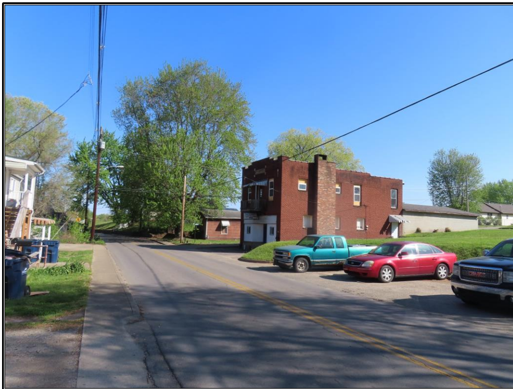
Figure A-45. Overview of KY 168 near its intersection with Sanders Road, looking north.
