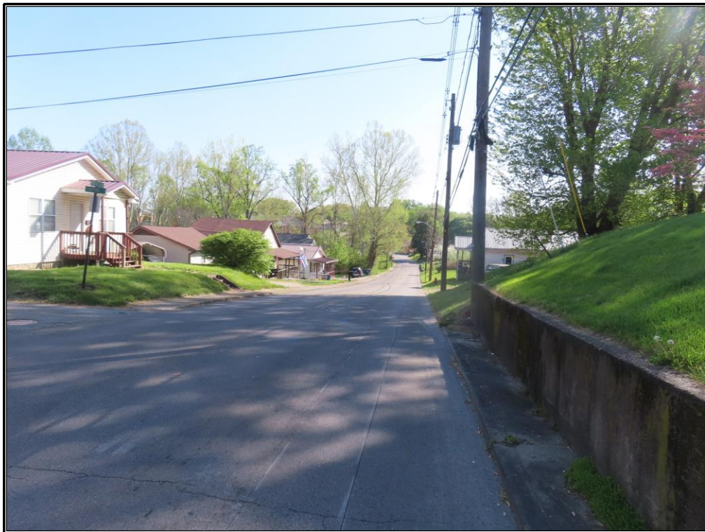
Figure A-44. Overview of Sixth Street near its intersection with Hinton Avenue, looking east-northeast.
