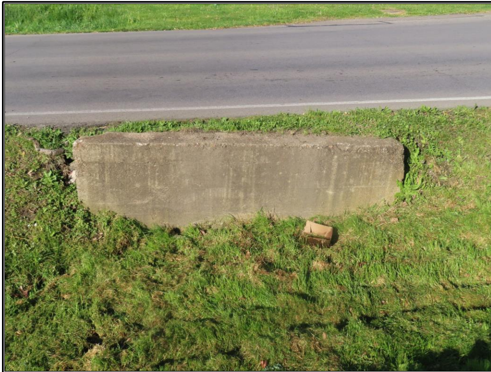
Figure A-23. CRA C: Pipe culvert's northeast headwall, looking west-southwest.
