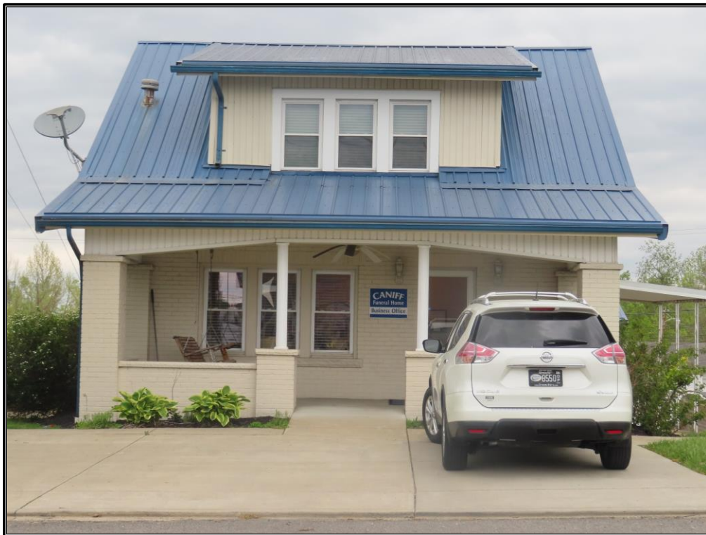
Figure A-12. BD 82: Façade of the converted residence, looking north-northeast.
