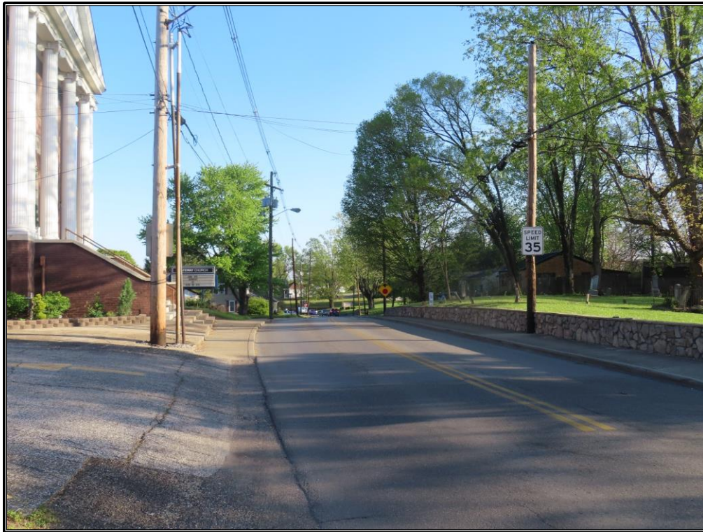
Figure A-7. Overview of the study area from the intersection of KY 168 and Dixon Street, looking north.
