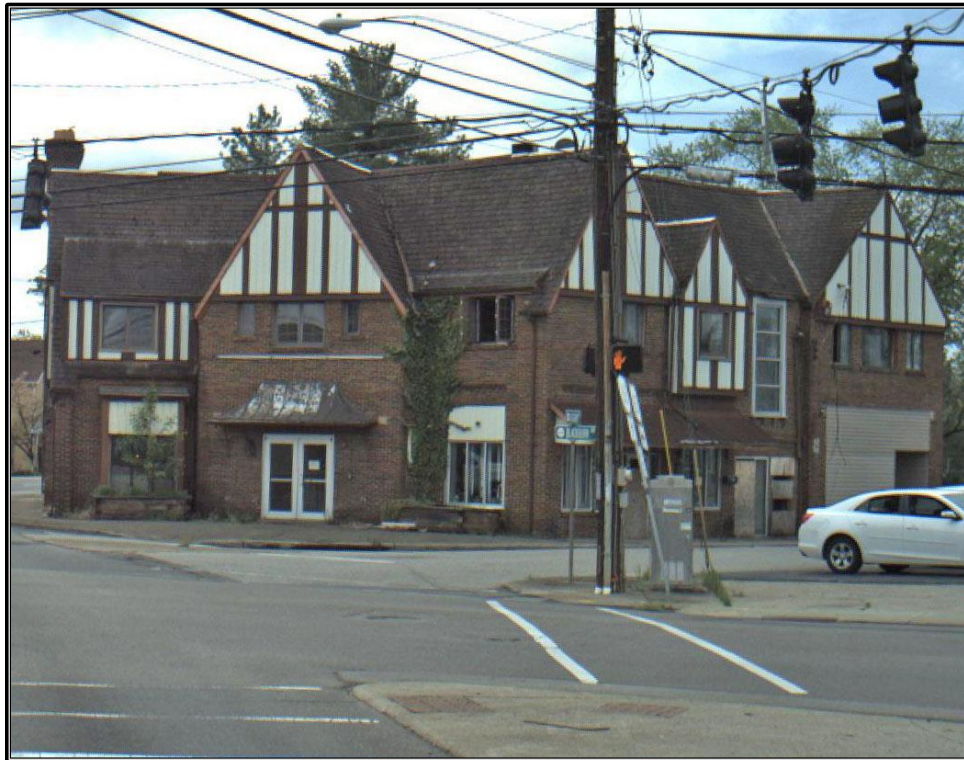
Figure A-34. CRA 1: April 26, 2022 view of the façade and northwest elevations of the building, looking west-southwest; from KYTC's Roadway Photo Viewer.
