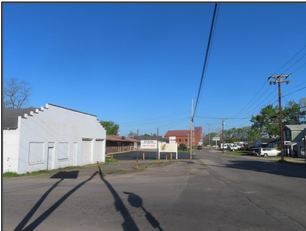
Figure A-38. Overview of KY 168 near its intersection with Main Street, looking west-southwest.
