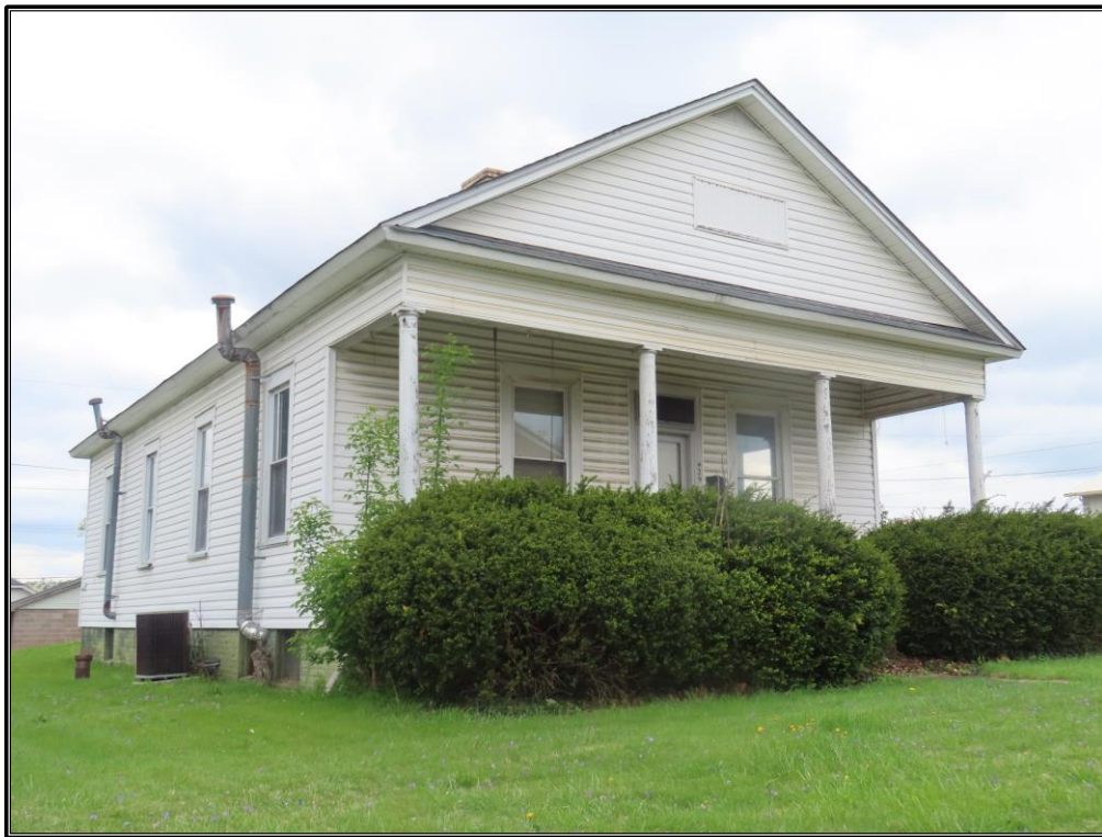
Figure A-19. BD 87: Southeast and façade elevations of the residence, looking west.
