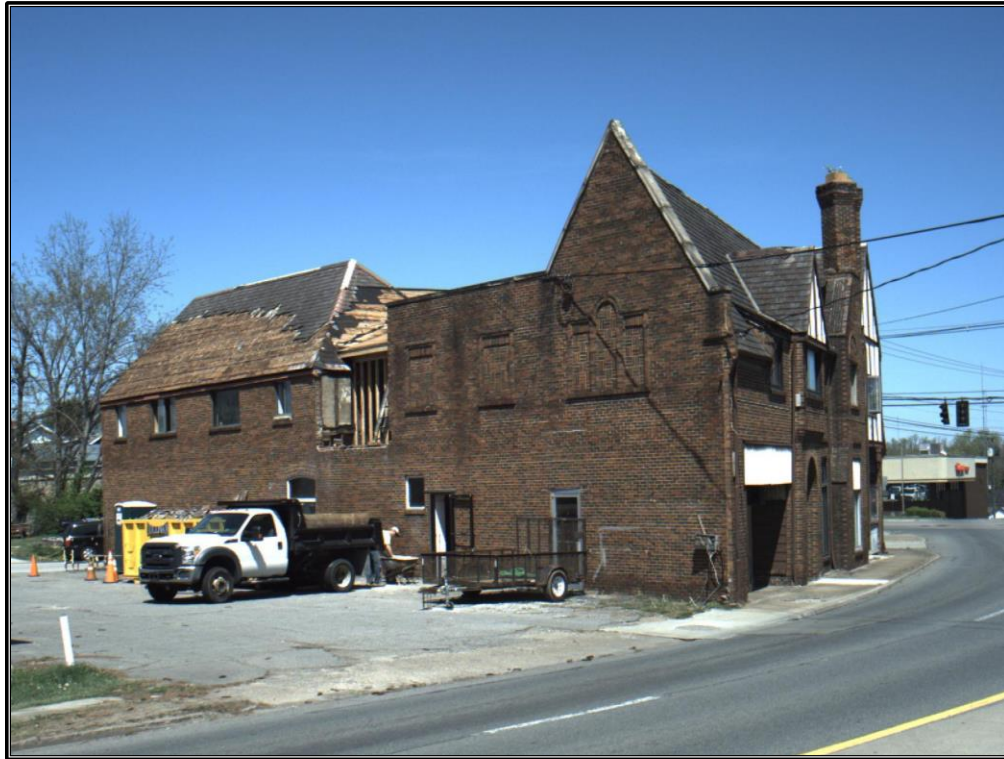
Figure A-37. CRA 1: April 10, 2023 view of the southwest (rear) elevation of the building, looking north-northeast; from KYTC's Roadway Photo Viewer.
