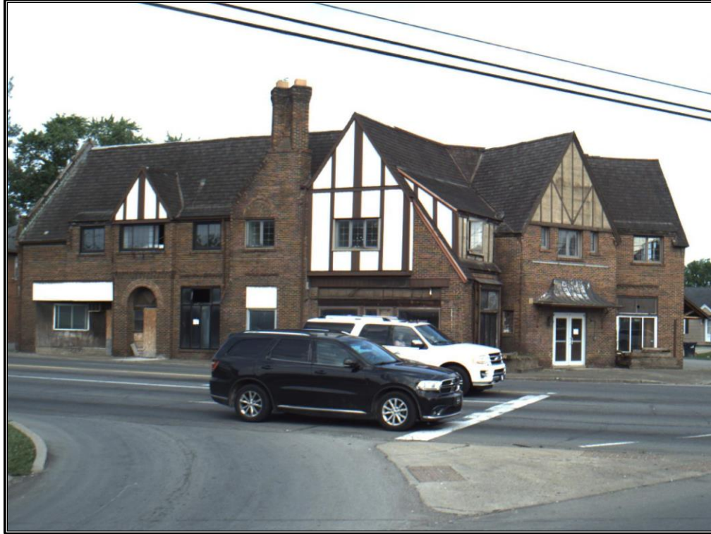
Figure A-35. CRA 1: April 10, 2023 view of the southeast and façade elevations of the building, looking northwest; from KYTC's Roadway Photo Viewer.
