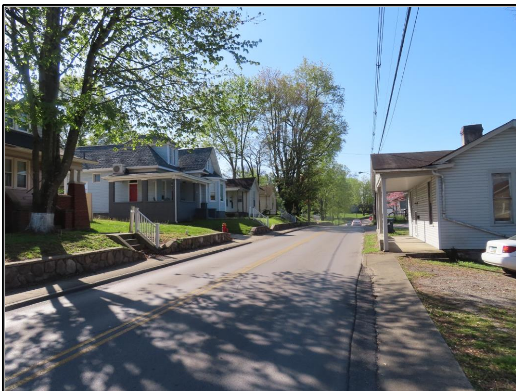
Figure A-46. Overview of KY 168 near its intersection with Sanders Road, looking south-southeast.
