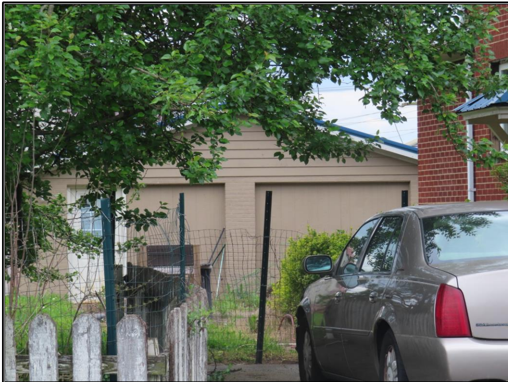
Figure A-16. BD 83: Associated garage (Resource B), looking west-southwest.
