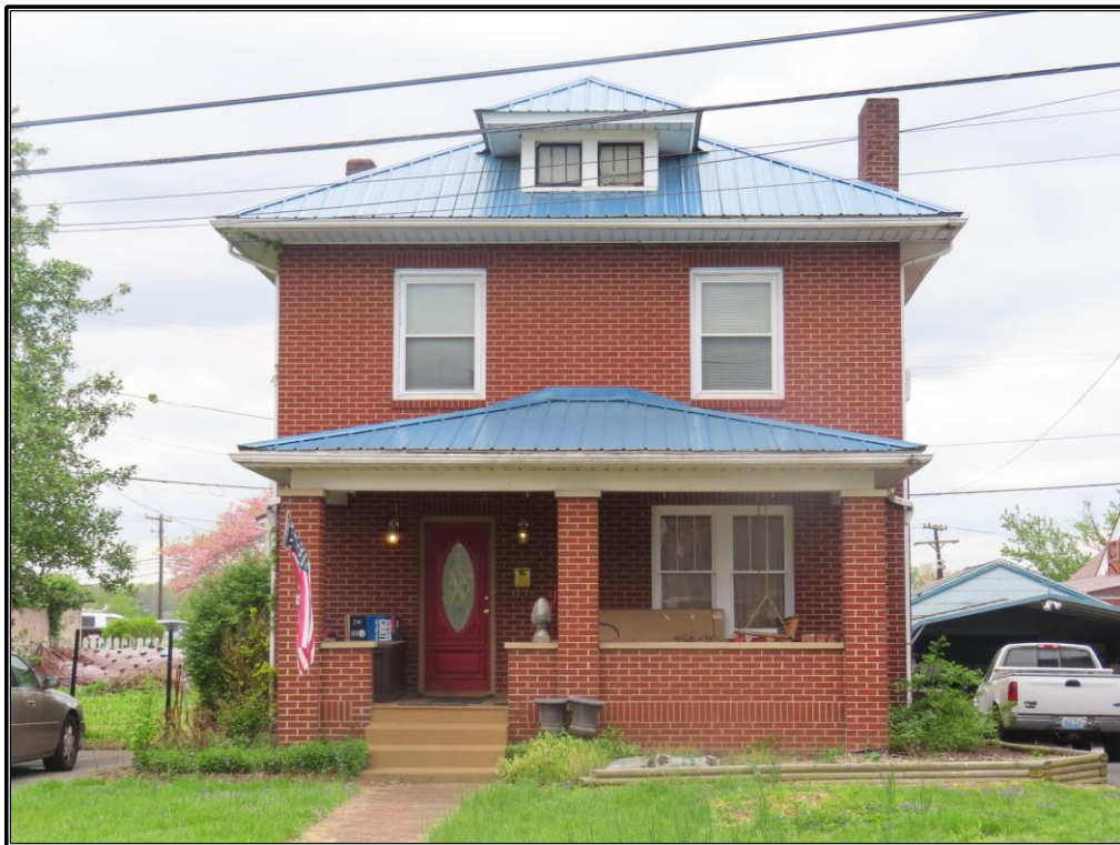
Figure A-14. BD 83: Façade of the residence, looking southwest.
