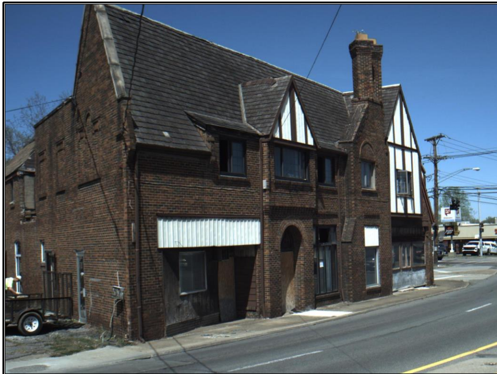
Figure A-36. CRA 1: April 10, 2023 view of the southeast elevation of the building, looking north; from KYTC's Roadway Photo Viewer.
