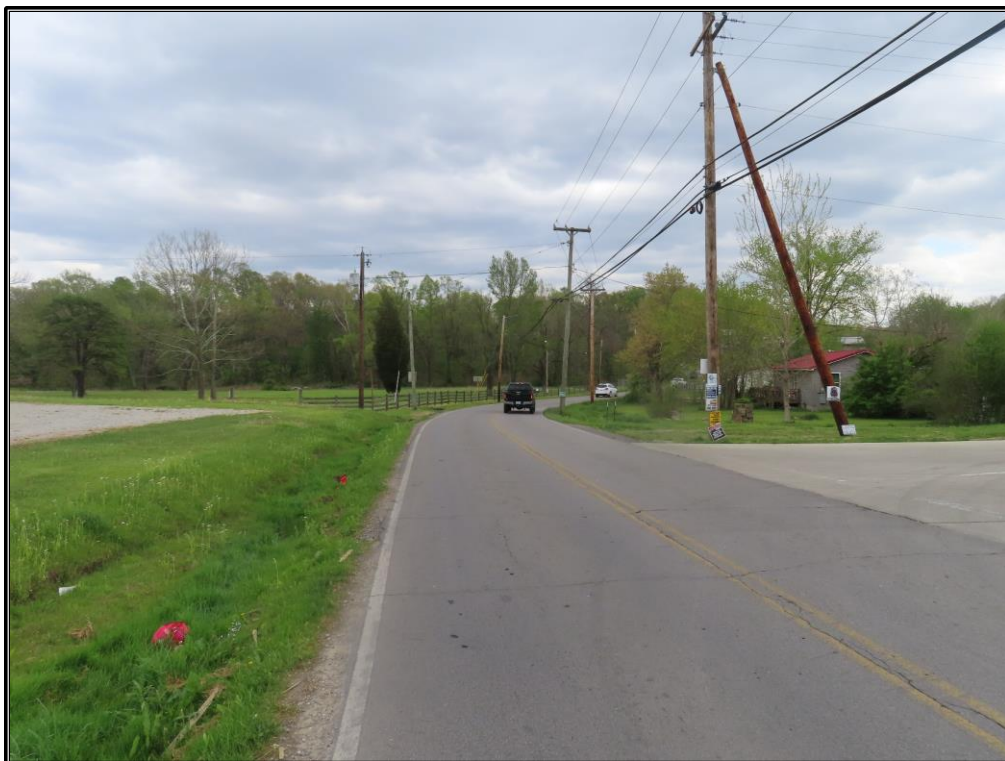
Figure A-4. Overview of the study area near the intersection of KY 168 and Kentucky Street, looking southeast.
